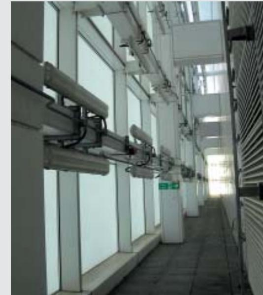
7. Crown lighting (at roof levels 43/44) for the HSBC symbol.
